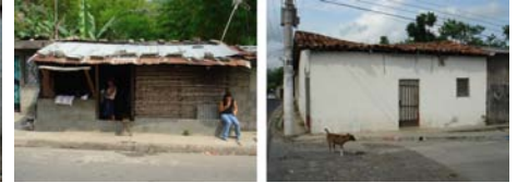
Figure 3. Typical bahareque buildings in rural areas.
