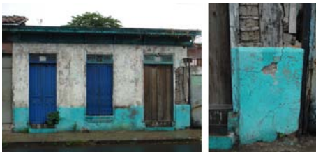
Figure 14. Bahareque building in an urban area with a pedestal made of clay bricks.
