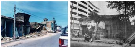
Figure 17. Damaged bahareque dwellings after the San Salvador earthquake on October 10, 1986 (left: San Jacinto neighborhood; right: after Kuroiwa, 1987). [Click to enlarge figures].
