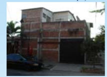
Figure 10. CLc - Confined claybrick masonry
