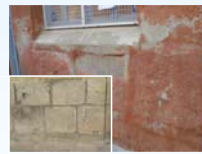
Figure 15. Pdc - 'Piedra de Canter' masonry of cut quarry stones, unreinforced
