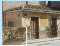
Figure 8. CC - 'Calycanto' (field stone, rubble stone masonry)
