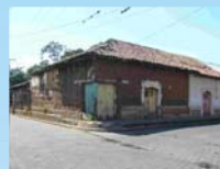
Figure 4. AD - Adobe brick masonry with adobe mortar
