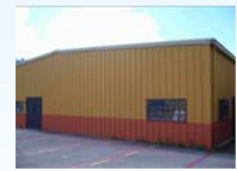
Figure 18. LT - 'Laminada Troquelada' steel frames with corrugated steel plates
