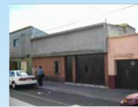
Figure 9. CLa - Unreinforced claybrick masonry
