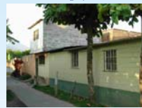
Figure 11. CBu - Unreinforced concrete blocks
