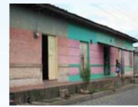
Figure 17. CBrc - Confined horizontal arrangement
