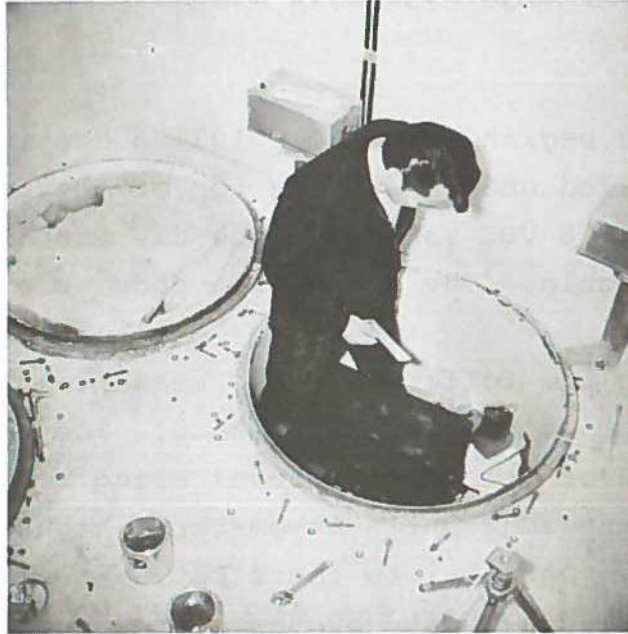
Figure 3.1 The NS and the EW tanks opened, the NS tank with insulating pads in.
