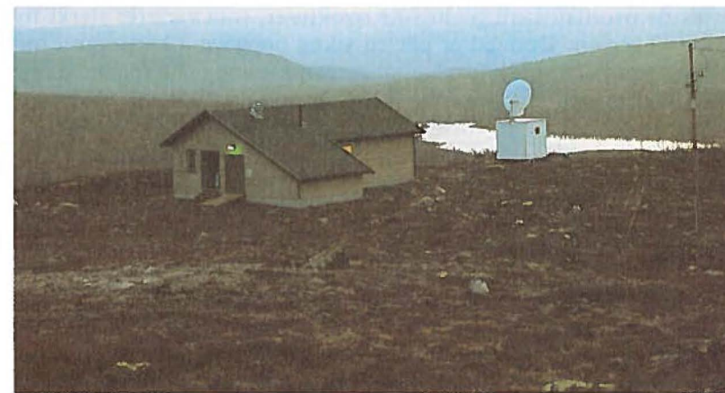
The ARCESS central field station houses instruments that provide power, timing signals and calibration commands to all instruments in the array. Data from the array seismometers are collected and transmitted by satellite to the NORSAR Data Center at Kjeller.
