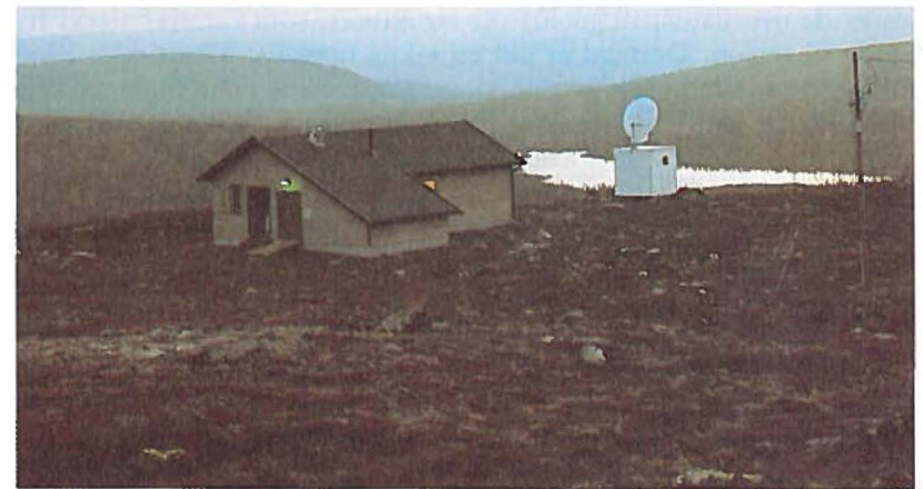
The ARCESS central field station houses instruments that provide power, timing signals and calibration commands to all instruments in the array. Data from the array seismometers are collected and transmitted by satellite to the NORSAR Data Center at Kjeller.
