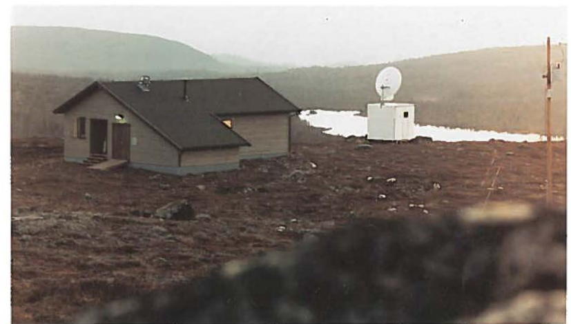
The ARCESS central field station houses instruments that provide power, timing signals and calibration commands to all instruments in the array. Data from the array seismometers are collected and transmitted by satellite to the NORSAR Data Center at Kjeller.
