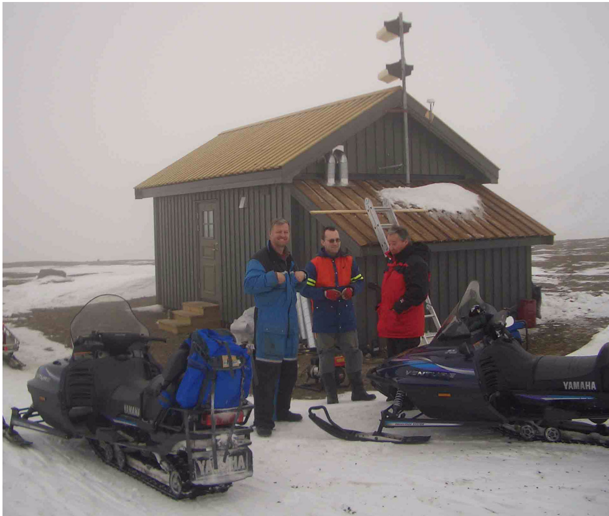
Fig. 4.4.1. The picture shows the new Spitsbergen array central hut located close to site SPB4, and was taken during installation of a new power support system in April 2004. The annex contains one tank holding 1000 liters of kerosene and one tank holding 1000 liters of water (with anti-freeze solution). The kerosene is used in the Sterling engines to heat the nitrogen gas, and the water is used to cool the gas. The heat transferred to the coolant is used for heating the hut.
