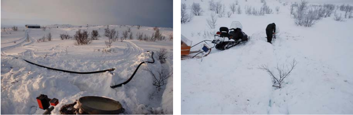
Figure 6.2.6. Burying the pipes.
