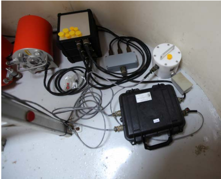
Fig. 6.4.4 NORES seismic and infrasound instrumentation, as installed in the field.
