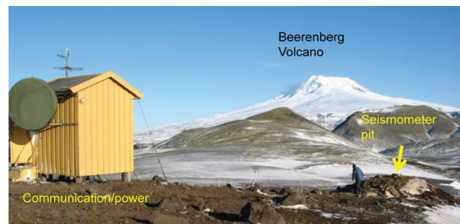
Fig. 10.2.2 The photo is from the JMJC site, showing the building for power and communications. The seismic vault is located to the right of the person. The Beerenberg active volcano is seen in the background.
