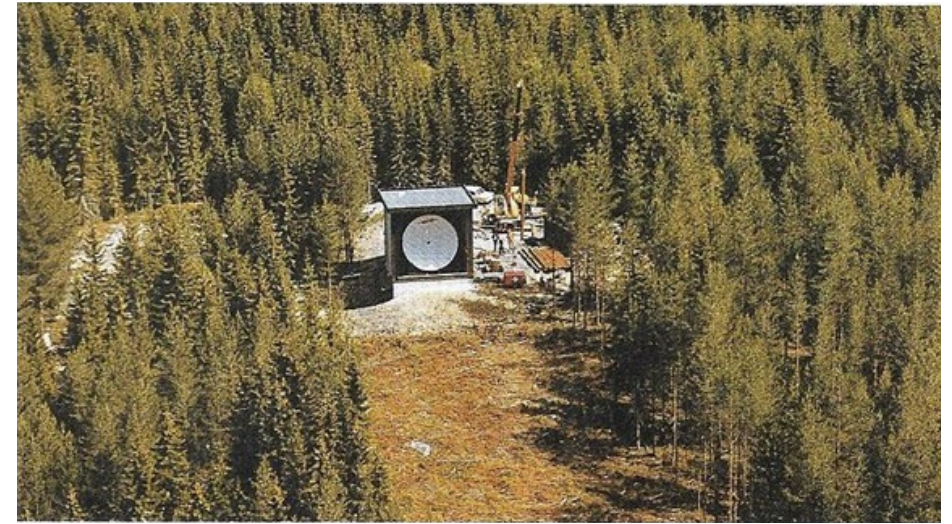
Fig 5.1.6 NORESS data were initially transmitted to the United States by satellite. A clearing had to be made in the forest to make the antenna visible to the low-elevation geostationary satellite. The original building was later rebuilt to house the Stendammen facility for equipment testing and experiments.
